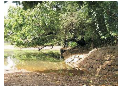
Bunds made of rocks constructed on one of the sides of the madaka to restrict the flow of water
