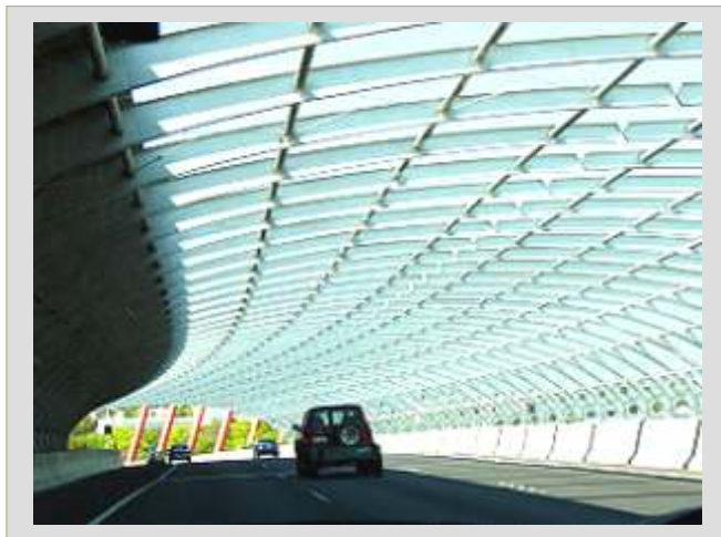
The sound tube in Melbourne, Australia, designed to reduce roadway noise without detracting from the area's aesthetics.
